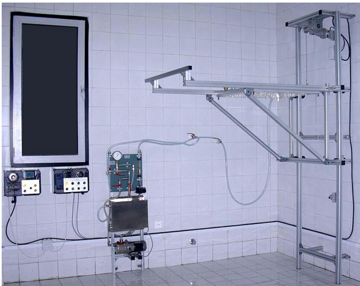
The photo shows the complete system, not only T1-37.
